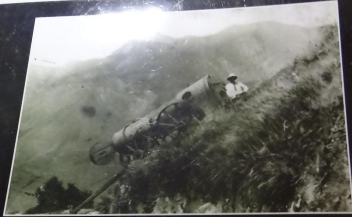
Tea Factory Boiler Manhandled up to Top Station c.1920
